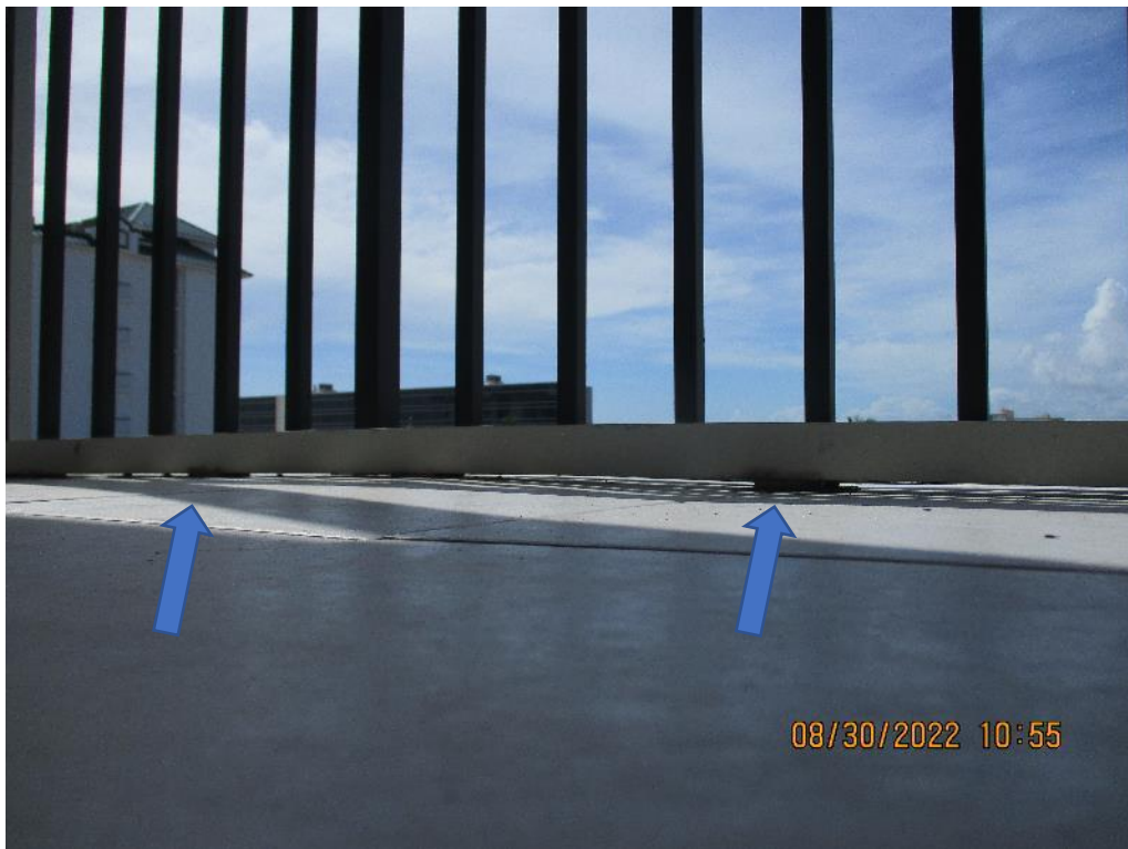
Shutter track with installed shims to promote positive drainage
