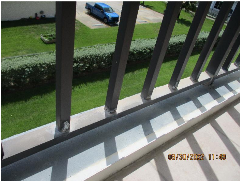
Railing deterioration
