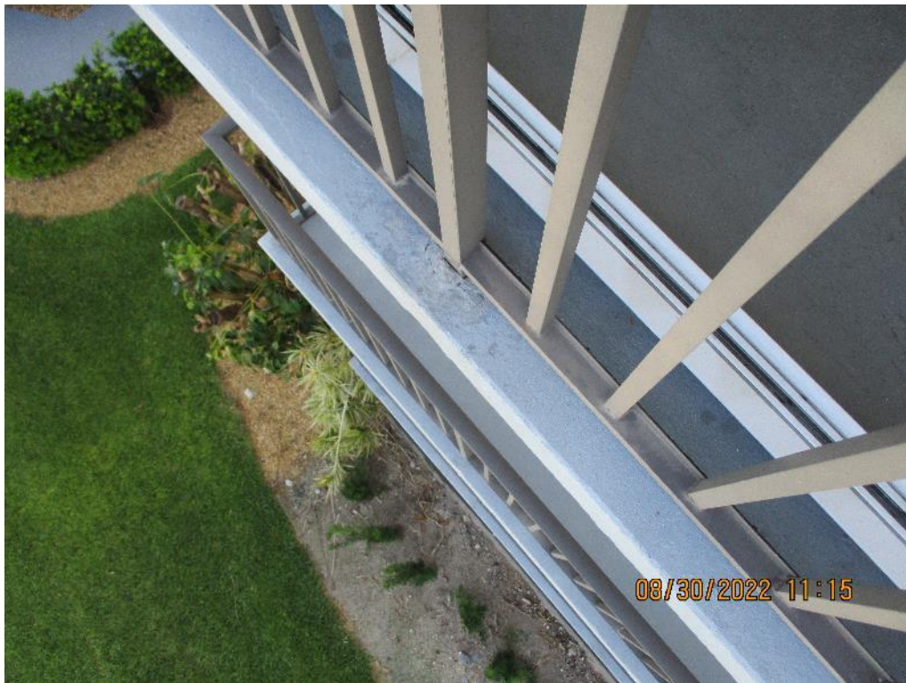
Example view cored railings
